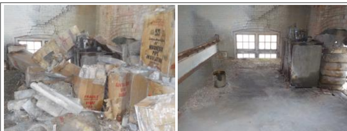
Before and after photos of asbestos storage area in main building. Photo credit: WWC Engineering
