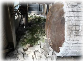
**Asbestos:** Significant volumes of friable and non-friable asbestos, some of it damaged, were identified. Examples include pipe insulation, plaster, building insulation, roofing tar and coatings, fire brick, linoleum, boiler gaskets, and pipe joints. Trace amounts of asbestos were found in soils outside of the building.
