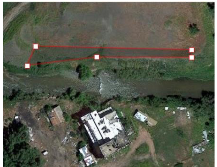
Figure 12: Approximate Solar Array Area
