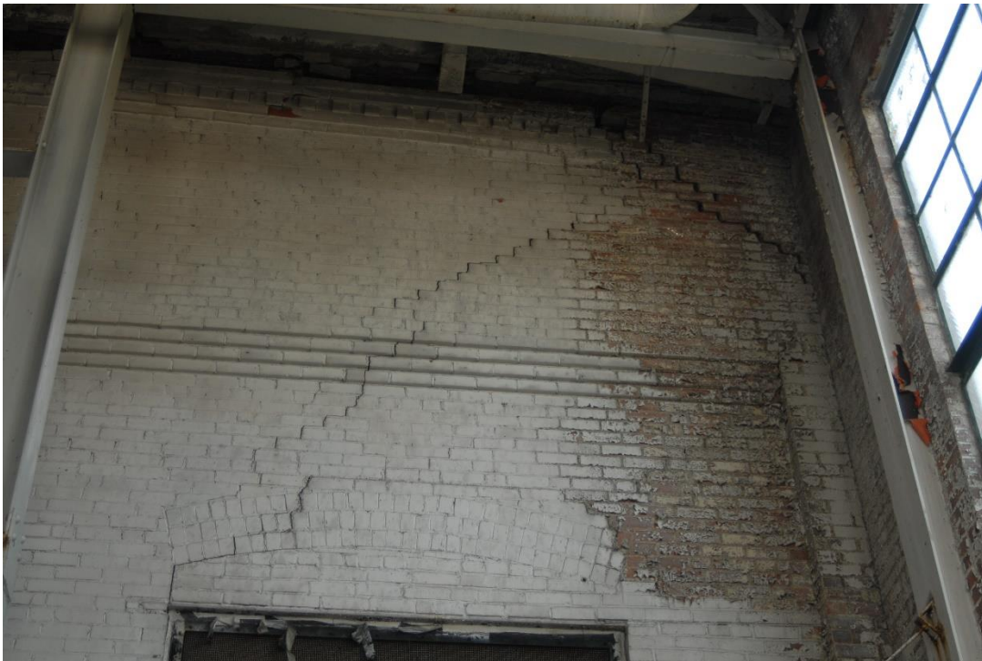
Photo 34: Crack in wall between 1950s and 1910 generator room, above doorway at east end of wall.
