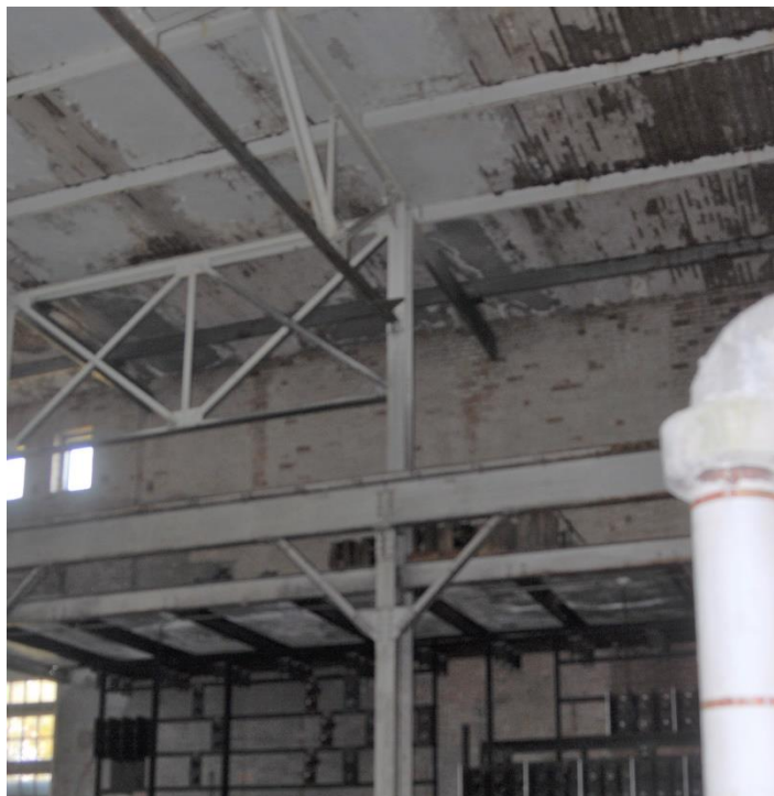
Photo 18: Steel column and trusses supporting roof and catwalk in 1910 building.
