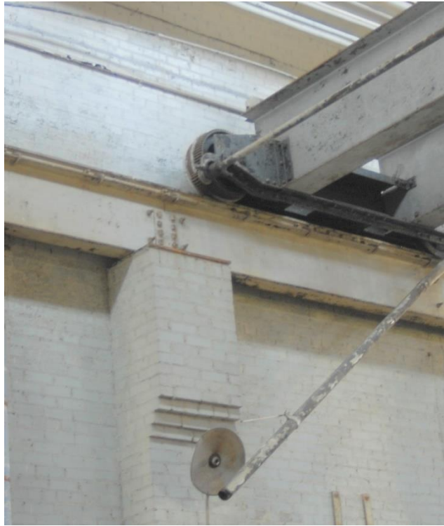
Photo 17: Crane rail supported on brick pilaster at center wall.
