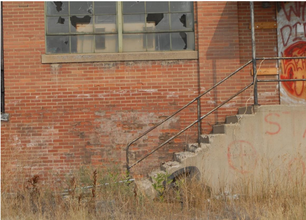
Photo 46: Spalled brick and damaged concrete stairs at south face of 1950s addition.
