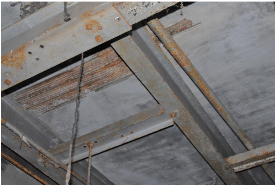
Photo 14: Underside of 1 st floor slab of 1910 building, showing “expanded metal diamond mesh” reinforcing.
