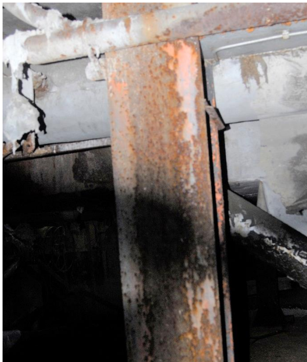
Photo 44: Column in 1950s basement, showing surface rust.
