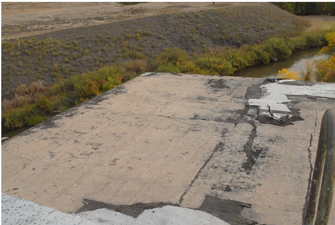
Photo 40: Worn, patched and damaged roof over office of 1947 addition.
