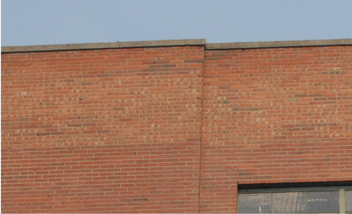
Photo 45: Past brick repairs at top of exterior brick in the 1950s addition.
