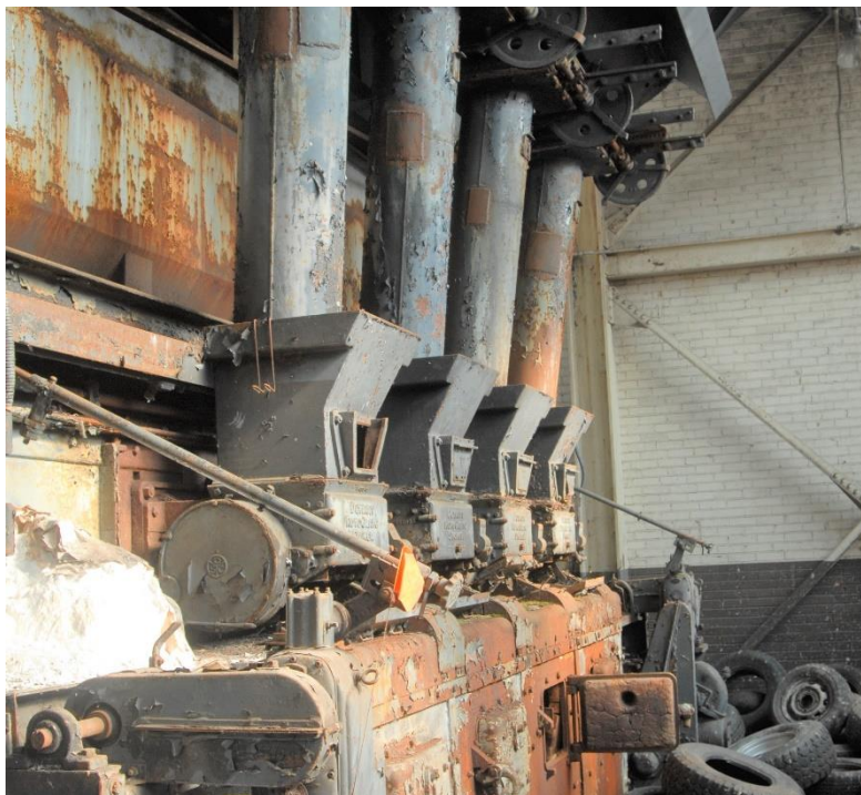
Photo 24: 1950s boiler room showing fireboxes and diagonal steel wall bracing beyond.
