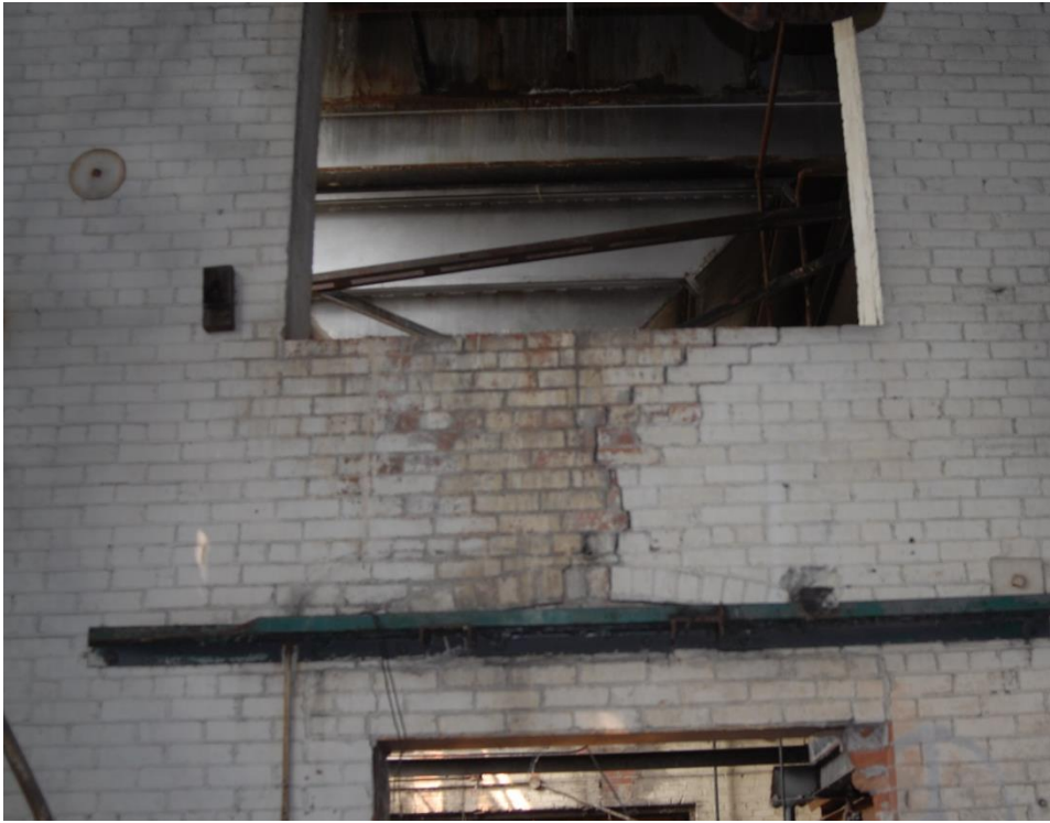
Photo 33: Crack in wall between 1910 & 1947 boiler rooms, above 1 st floor doorway.
