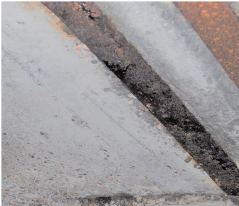
Photo 28: Deteriorated bottom flange of steel beam that spans across ash tunnel and supports tunnel roof.
