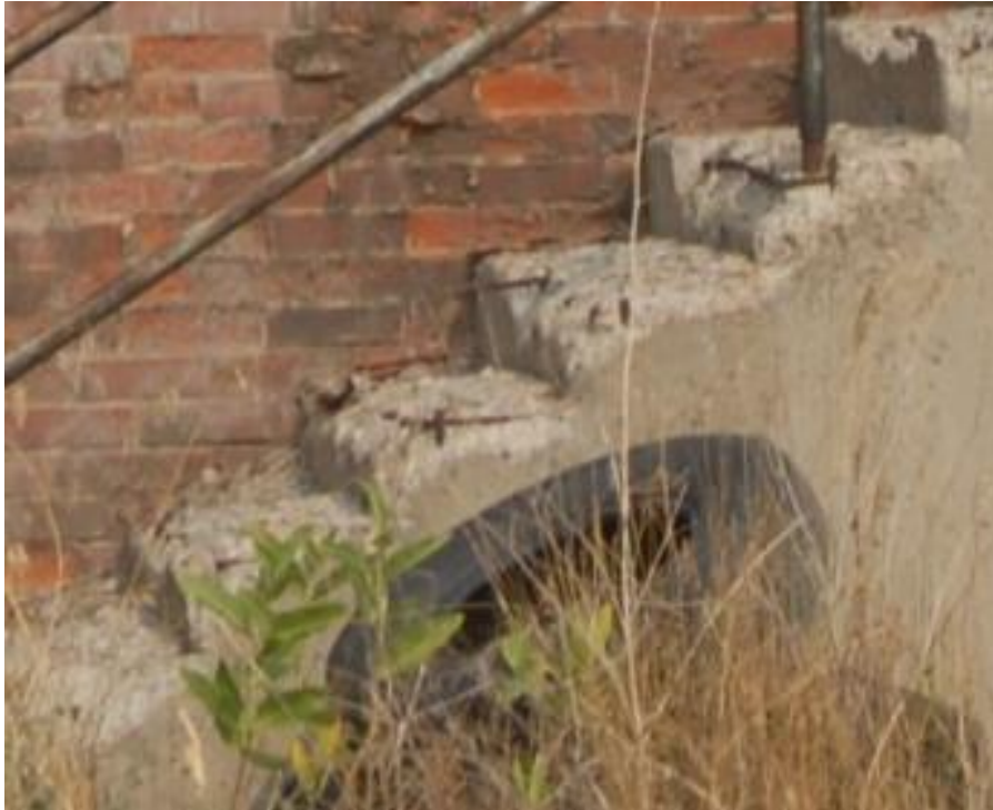
Photo 47: Close-up of damaged stair treads at south face of 1950s addition.
