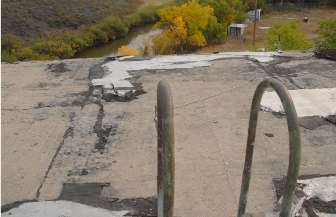
Photo 39: Worn, patched and damaged roof over generator room in 1910 building.
