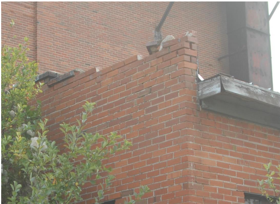
Photo 48: Damaged north parapet at small ancillary building
