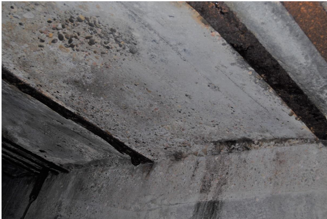
Photo 12: Ash tunnel roof showing river rock aggregate and shallow arched slab.
