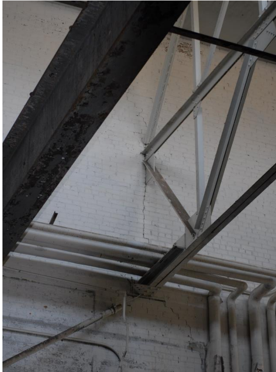
Photo 31: 1910 roof truss diving into center wall, with crack between top and bottom chords of truss.
