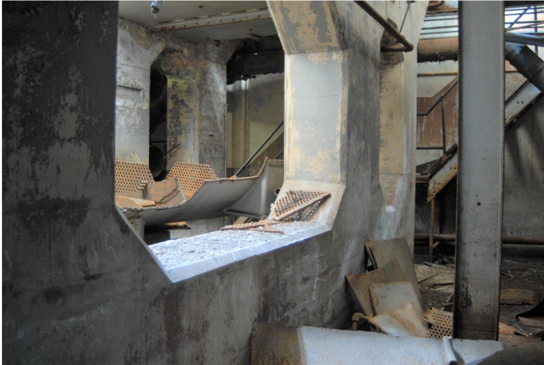
Photo 13: Basement of 1910 building, showing large concrete pillars supporting generators, and steel column.
