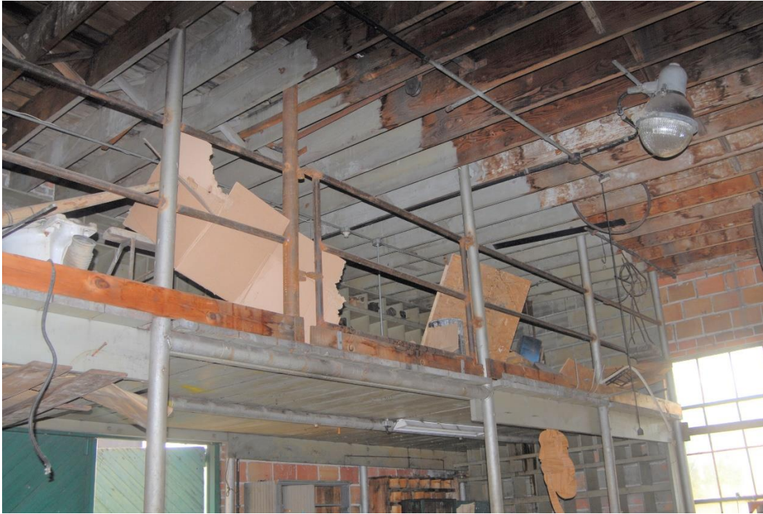
Photo 27: Ancillary building interior, showing mezzanine and wood roof joists.
