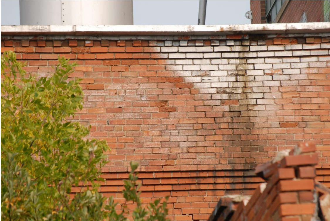
Photo 37: Damage to top five feet of 1910 building.
