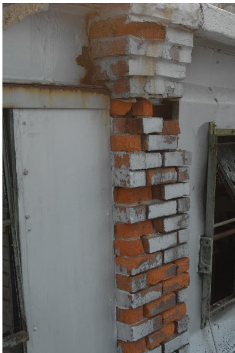
Photo 42: Damaged brick pier at clerestory of the 1947 addition.
