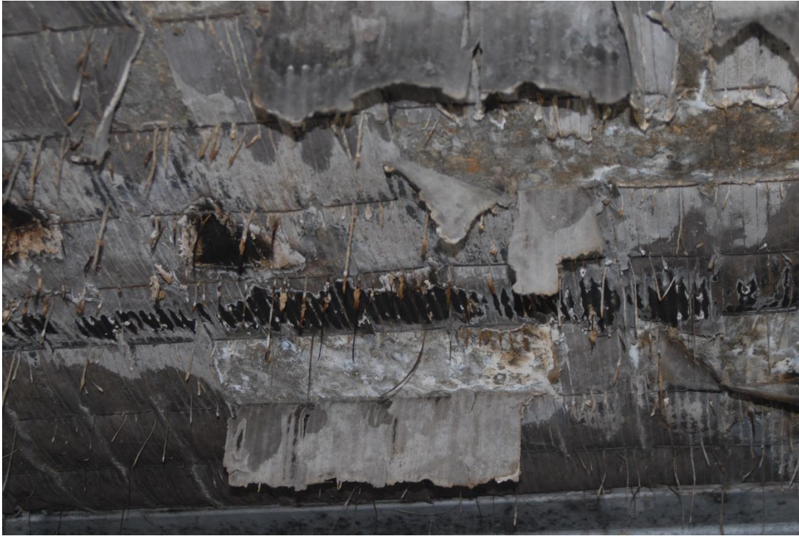
Photo 41: Fibrous material and wire mesh hanging from clerestory roof ion 1947 addition.
