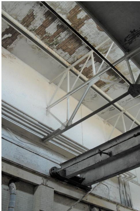
Photo 16: Trusses in 1910 generator room, supporting roof and supported on center wall.
