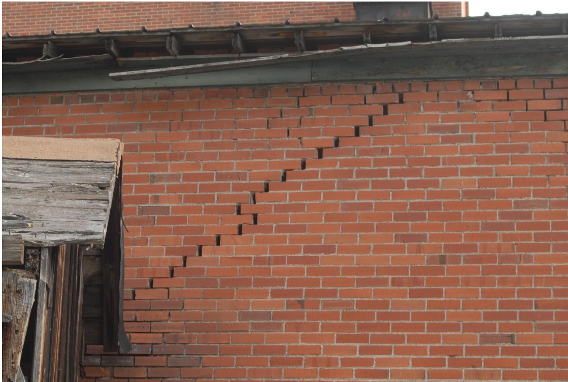
Photo 49: Crack in west wall of ancillary building, resulting from settlement of the southwest corner of the building.
