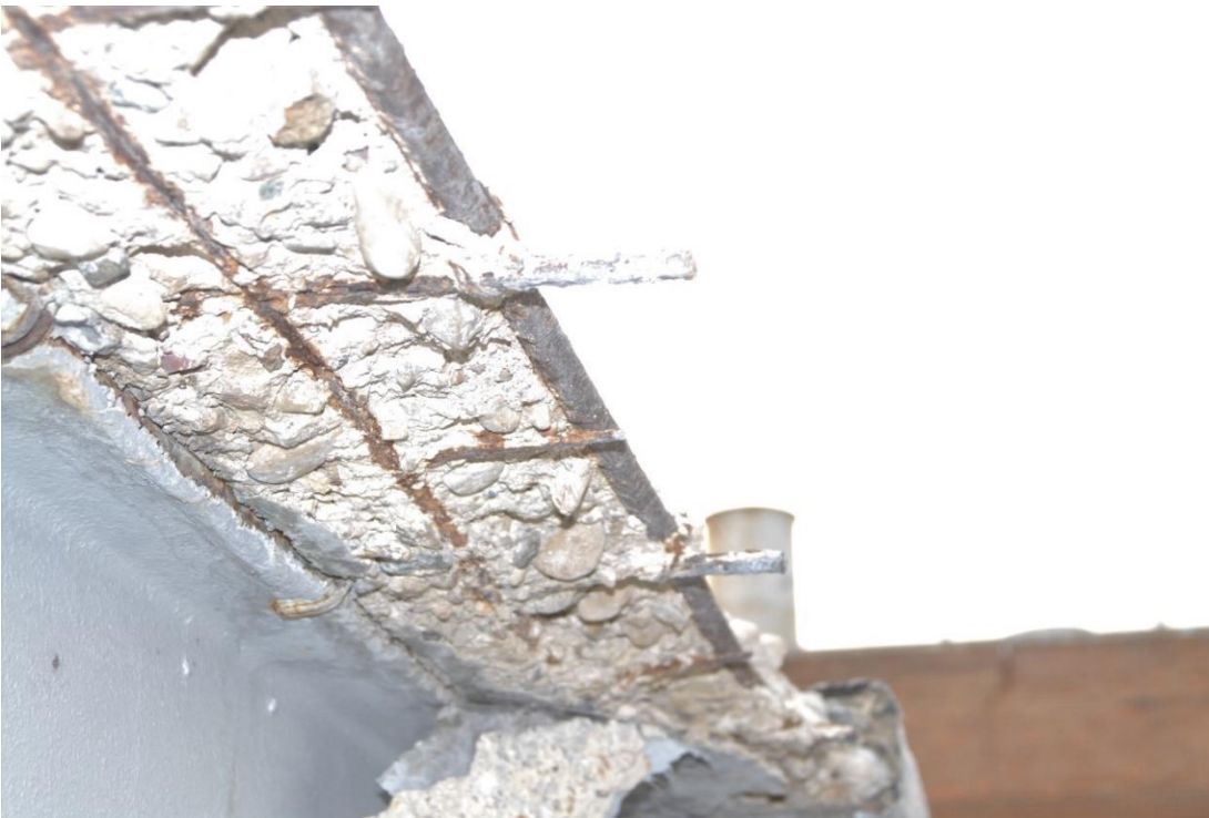
Photo 30: Deteriorated roof edge of 1910 clerestory roof – concrete has fallen away, leaving only reinforcing bars.
