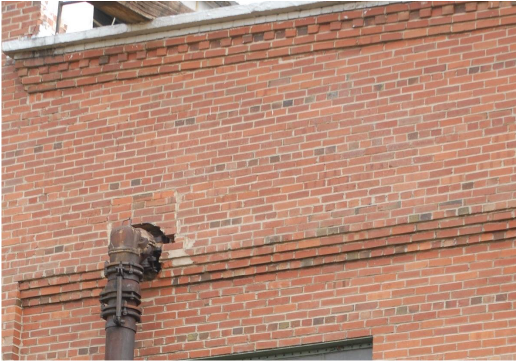
Photo 15: Decorative brick above windows and at top of wall of 1910 building.
