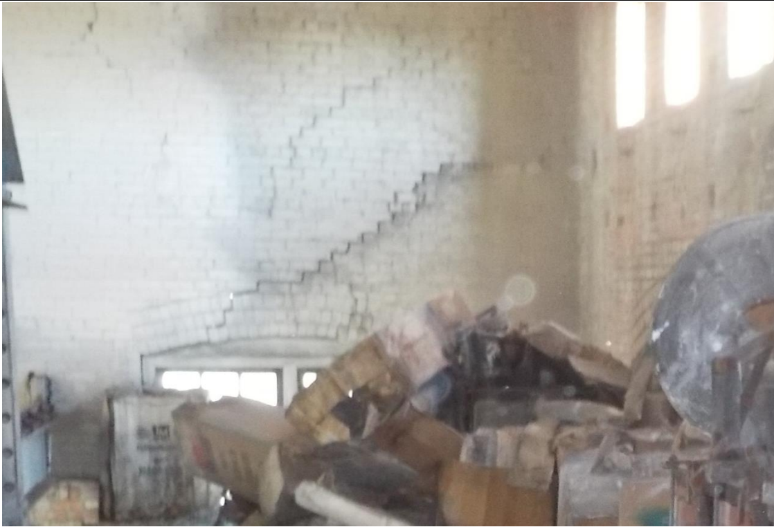
Photo 35: Crack in north wall of 1910 building, at east end, above mezzanine.
