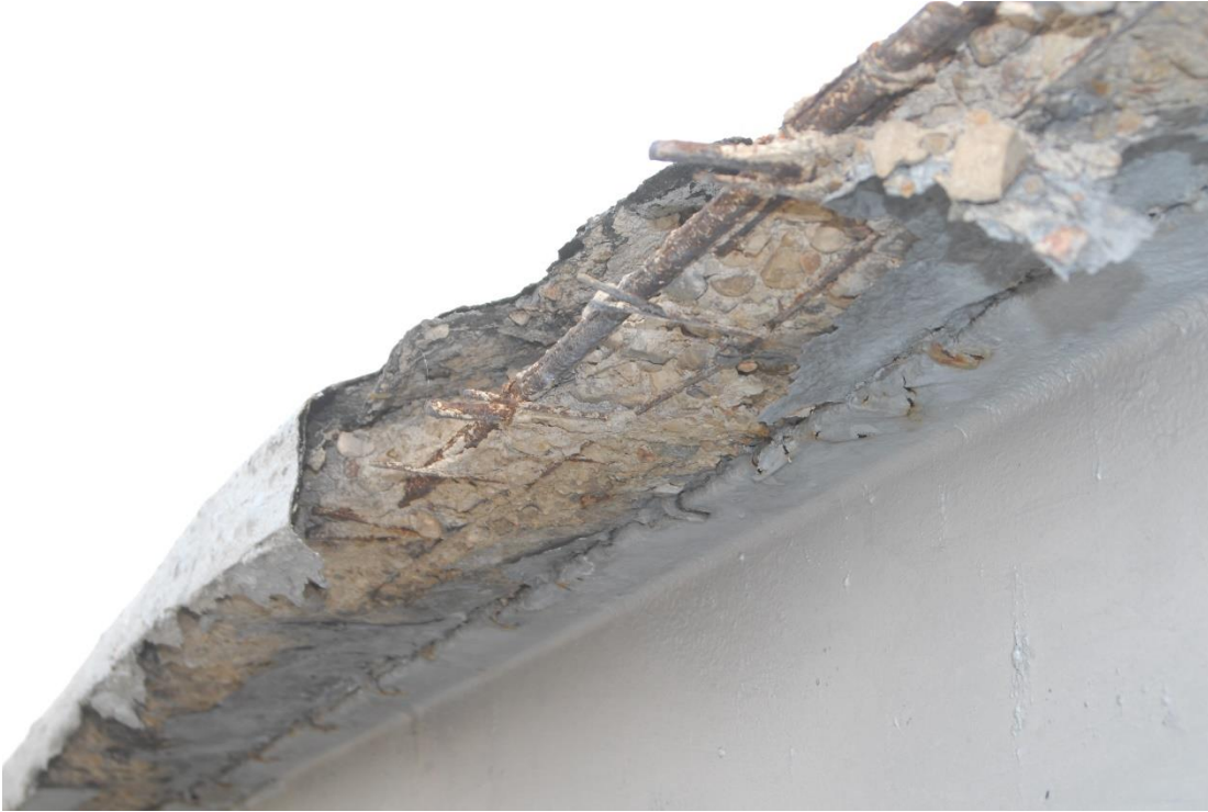
Photo 29: Deteriorated west edge of 1910 clerestory roof.
